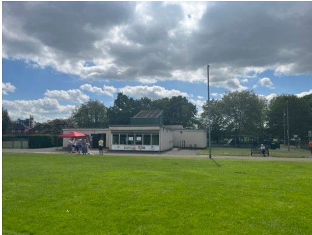
Existing pavilion to be demolished
